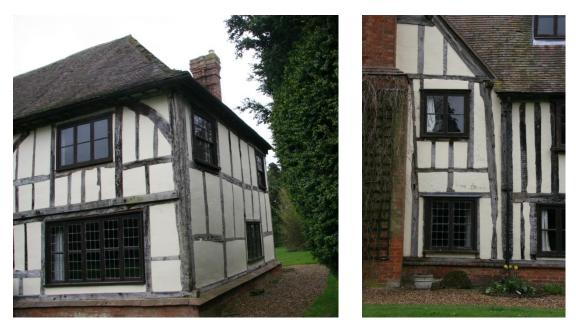
Figure 6: The second medieval hall (left) and (right centre) the corner posts of the two frames, side-by-side.
