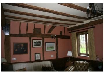
Figure 10: Oak framing inside the 'solar'
